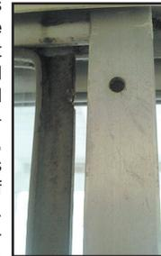
producing a sort of pregnant look around the area where the wheels live inside the rail. This "Pregnant Door Syndrome" will, in time, cause pitting and completely "eat" up the aluminum frame in this area. Once this occurs, the door is a candidate for replacement. If caught in time, this can be repaired, although this situa-
