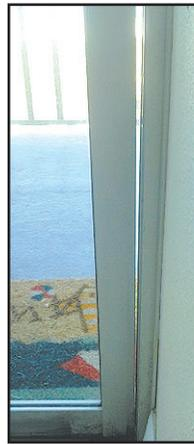
it is NOT the end of the door's life! Glass separation is generally an indicator of additional problems in the door, one of which is that the screw systems need reinforcement. We kidding-ly tell our clients that we're the company out there who will "screw you" and you will appreciate it! However, corroded screws are just a part of the problem. Fixing this problem requires deli-
